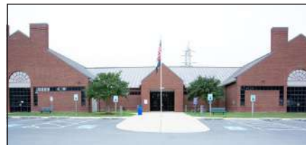
LOCAL 4 Commissioners discuss renovations for Charlotte Hall Library
