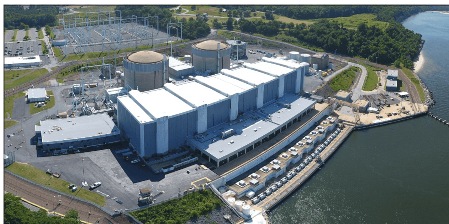
Calvert Cliffs Nuclear Power Plant
