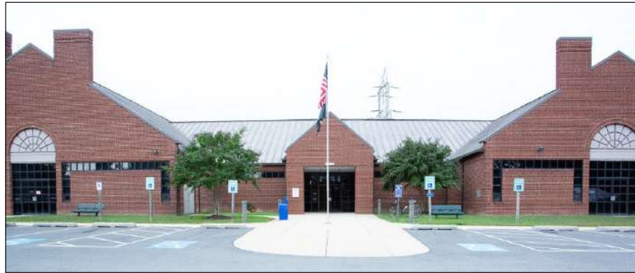
Charlotte Hall Library is currently on the left and SMRLA is on the right.
